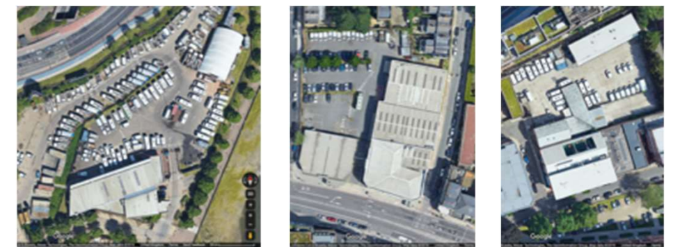
PVs on all large Council buildings' roofs – for example, the transport / depot sites have significant roof areas, and potentially car park areas, which lend themselves well to large PV installations: Vehicle Testing Station, Blackwall (left); Car Pound (middle); Toby Lane depot (right).
