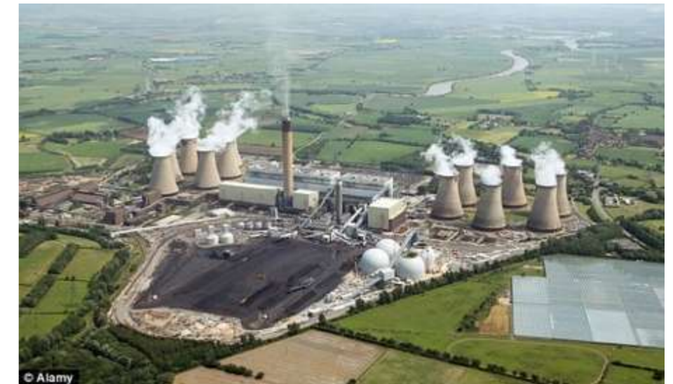
DRAX Power Station is operating a Bioenergy with Carbon Capture and Storage pilot project, capturing just 1 tonne of CO 2 per day.
