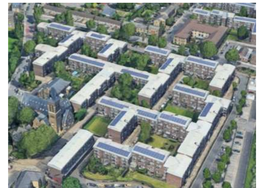
Housing blocks in Tower Hamlets already include significant PV installations
