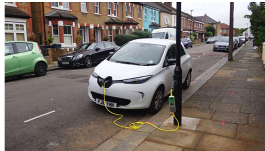
An electric vehicle charging point integrated with a lamp post on a UK street. Chargers that do not offer debit/credit card payment should be avoided if possible, as these may be phased out by legislation.
